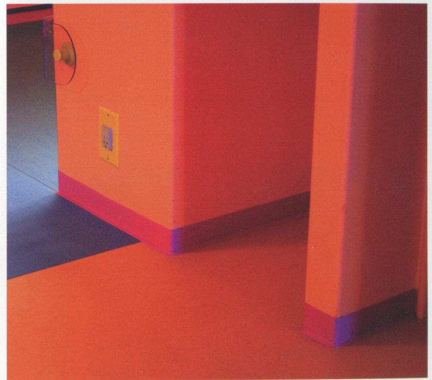
A total of 65 kilometers of pink-coloured rubber floor-moulding was especially produced for the hospital.
